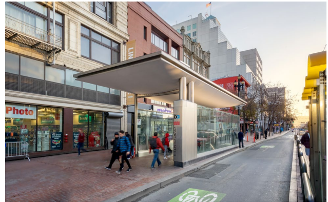
The Completed Powell Station Prototype Canopy
