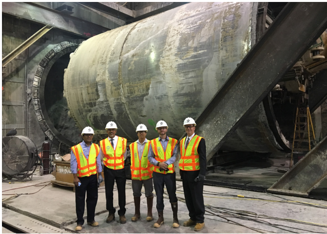
Steve Kappler joins project team members to view the tunnel boring machine launch on LACMTA's Crenshaw/LAX Transit corridor project.
